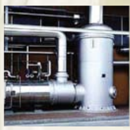
Sulfer Burner with Heat Recovery Steam Boiler
