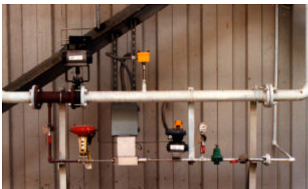
Figure 4. Ammonia/Air Distributor
